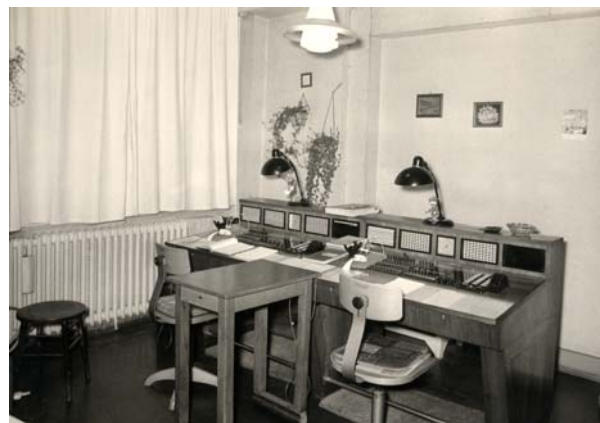
Switchboard at the Hanover branch, circa 1960
