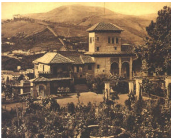
Torre de las Damas – Gwinner's erstwhile country estate in the Alhambra complex
